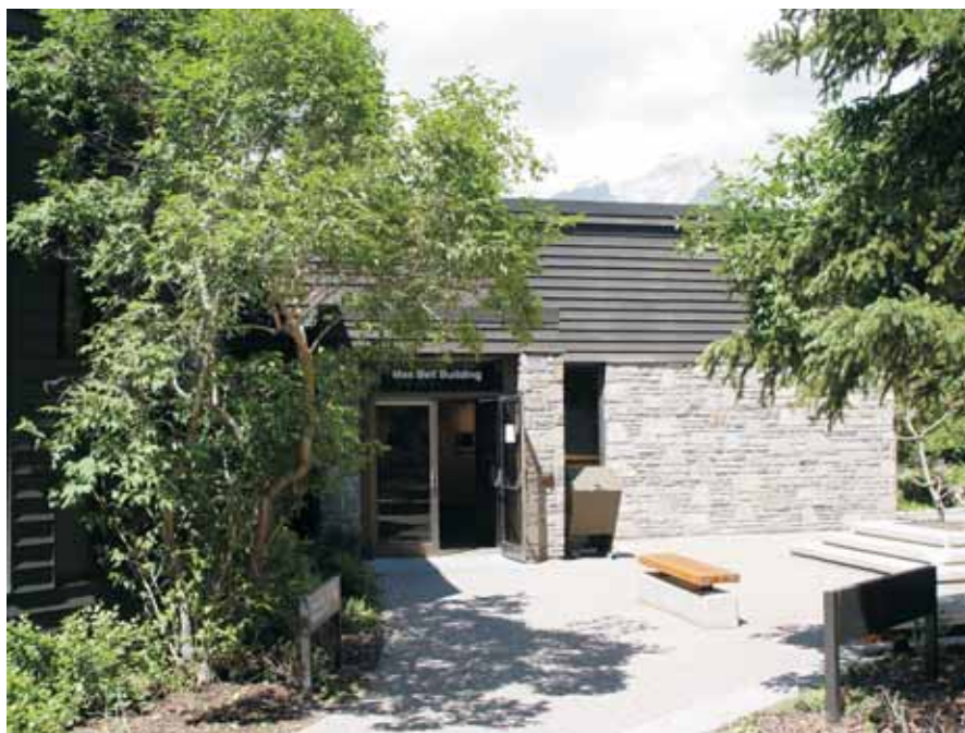
Max Bell Building at the Banff Centre.
