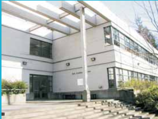
East Academic Annex, PIMS-SFU Site Office.
